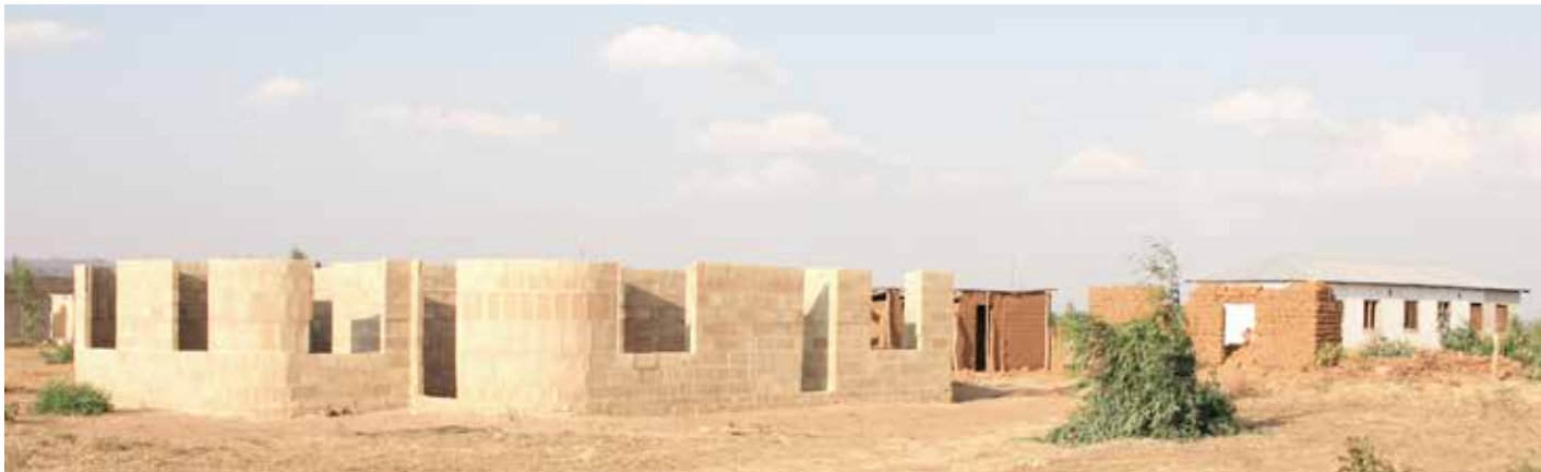
Image 10: Those who can afford it, tend to build with locally produced concrete adobe bricks.
